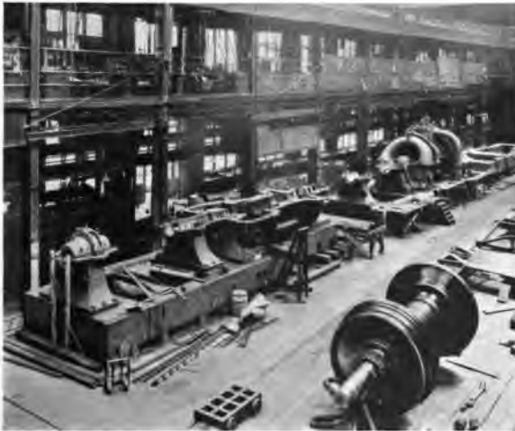
Assembling 7,500 HP Turbines for Testing
